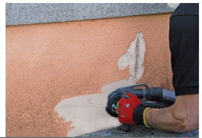
PCD milling disc for concrete surfaces (P/N 37125)
